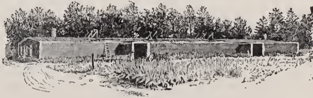
2404. A half-cellar storage.
